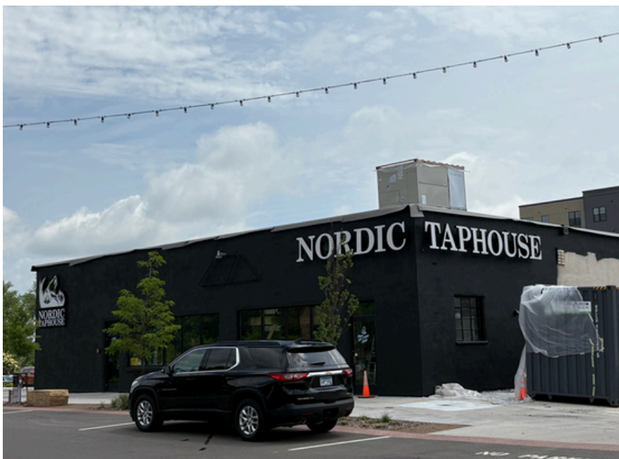
Photo of Nordic Taphouse (under construction), City of Monticello
