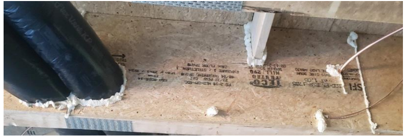
Example of draft stopping of floor truss.
