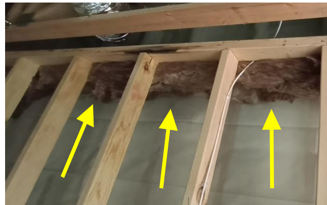
Example of fire blocking of furred out wall and ceiling using batts of insulation.
