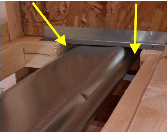
Examples of fire blocking needing to be added between the wall and ceiling.
